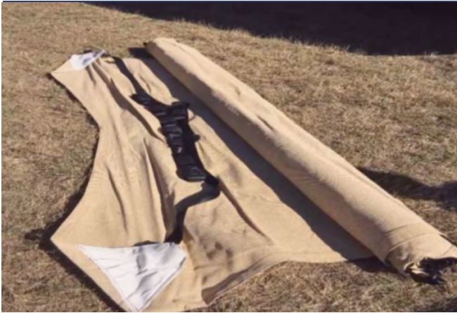
1) Complete "Assembly Instructions" prior to installation. Roll up canopy with fiberglass installed.
