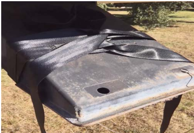
3) Install (2) 12' anchor straps in front of RV. Notice "criss-cross" pattern.
